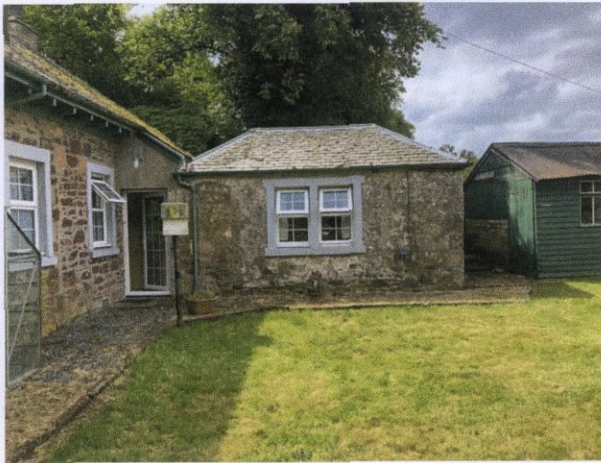
View of existing extension and shed.
