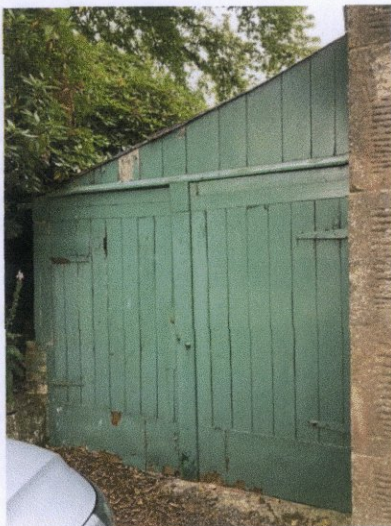
View of garage/ shed on gable.
