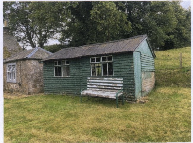
View of existing shed.
