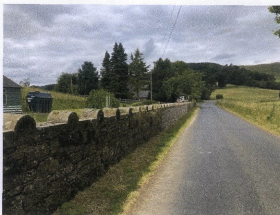
View down road where new parking access to be formed.
